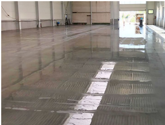
Application in the construction industry for sealing (Sailer Markus GmbH, 2022)
